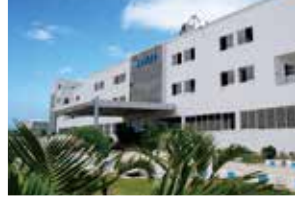
Rudrapur Plant (Green Building)
