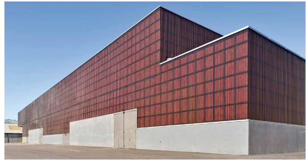
▲ External facade in accordance with Minergie standard
