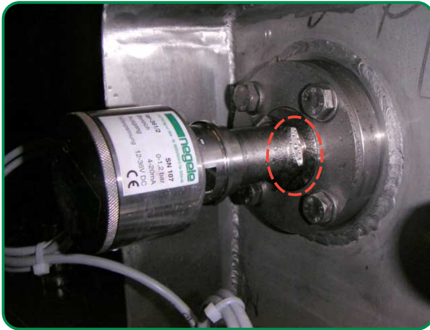
Pic.1: Condensation at the level sensor LAR-361
